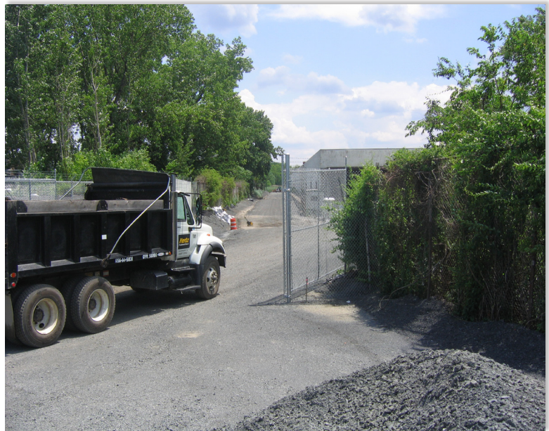
A project dump truck enroute from the storage site to the Sears warehouse property (in background).
