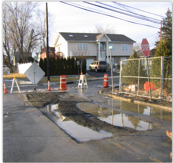
The nearly-completed water line repair site next to a designated Maywood Site vicinity property (inside fence).
